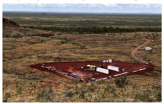
**Figure 12**. Exploration camp construction underway with levelling and compaction of 70m x 70m area in preparation for dome-sheltered core yard, accommodation, ablution block, workshop and offices. The prominent hill in the background is the western part of the Main Hill deposit. View looking southwest.
